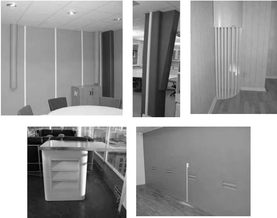
Figure 5.23 Some of the impinging jet terminal devices that are in use (courtesy of Air Innovation, AB).
