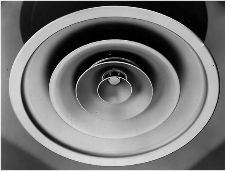
Figure 5.12 A multi-cone ceiling diffuser.
